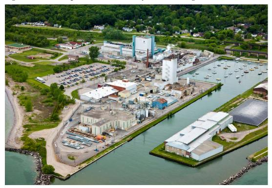
PHCF primarily converts uranium trioxide (UO<sub>3</sub>) powder produced by Cameco's Blind River facility into uranium dioxide (UO<sub>2</sub>) and uranium hexafluoride (UF<sub>6</sub>). UO<sub>2</sub> is used in the manufacture of CANDU reactor fuel (natural uranium), while UF<sub>6</sub> is exported for further processing before being converted into fuel for lightwater reactors.
